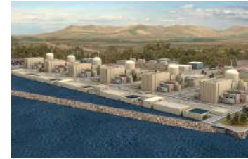
EPR JAITAPUR The world largest nuclear power plant 6 units, 9.9 GWe
