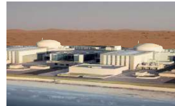
EPR KSA PROJECT 2 EPR Units
