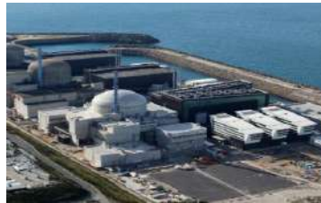
EPR FLAMANVILLE 3 The first EPR unit built in France
